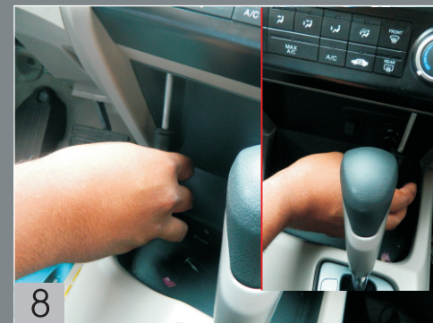
8 Take out the two fixed screws of cigarette light below the original CD host.
